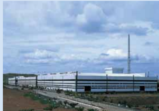
Jain Food Processing Plant at Jalgaon, India
