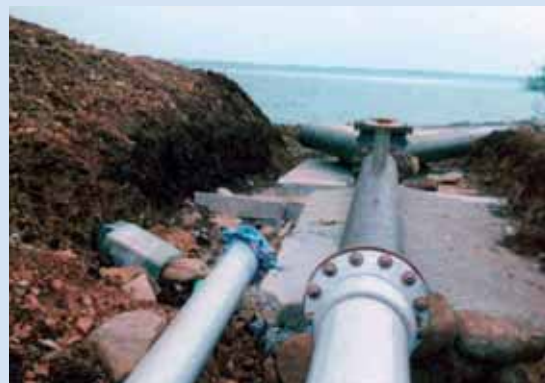
Jain HDPE Effluent Sewerage line installed under the sea
