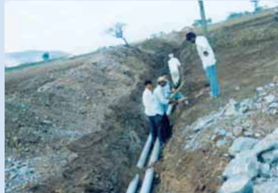
P.E. drinking water pipe being laid
