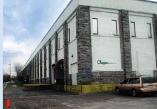
Jain Micro-Irrigation Plant at Watertown, USA
