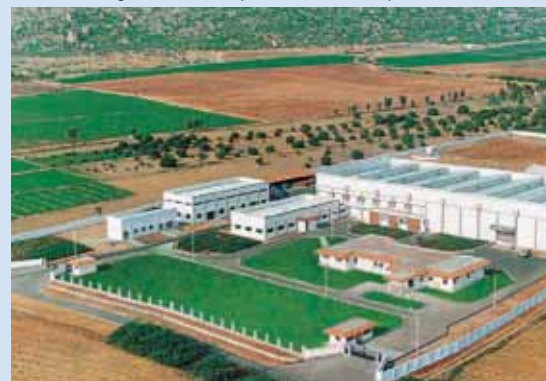
Jain Micro-Irrigation & PVC Pipe Plant at Udumalpet, India
