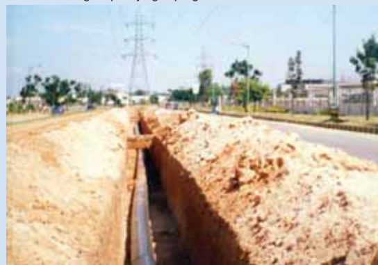
HDPE Sewerage Pipe laying in progress
