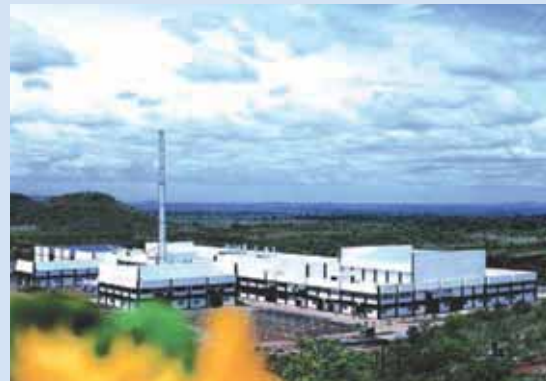
Jain Food Processing Plant at Jalgaon, India
