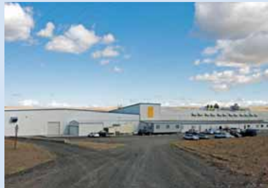
Jain Food Processing Plant at USA
