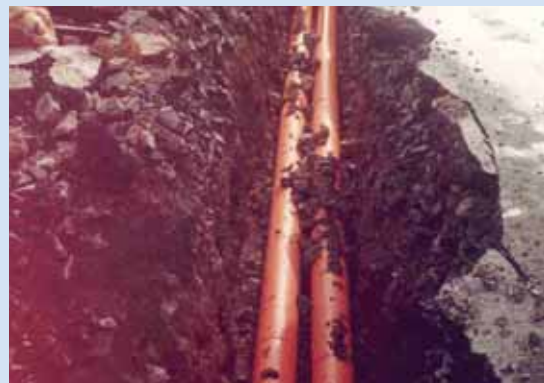
P.E. fibre optic cable installation
