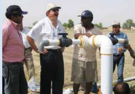
Field installation of PVC pipes & fittings at a site in Africa
